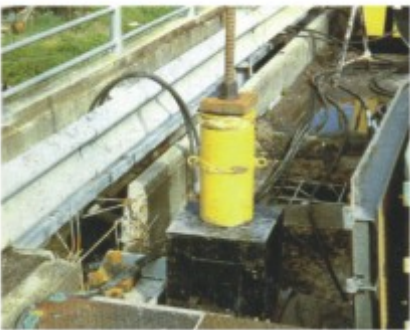
图 为双作用中空柱塞油缸 用于调平桥面。 The picture shows the use of double -acting hollow plunger cylinders in leveling the bridge deck.
